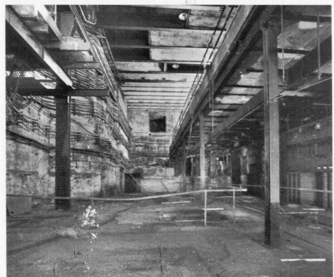
Embankment former substation. Photo Nick Catford
